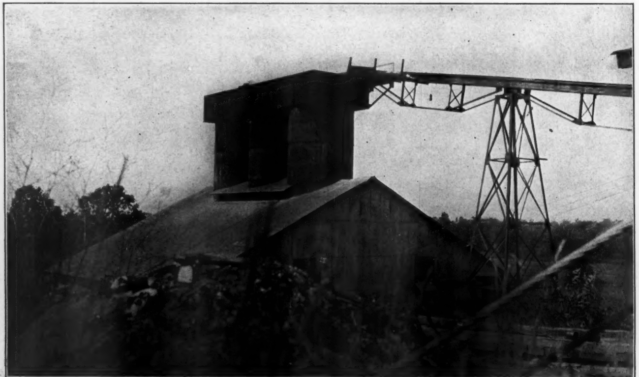
View of Steel Kilns with Steel Trestle Leading to Top
